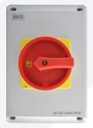
On the underside of the inverter the DC switch needs to be reset to allow the energy produced by the panels to continue to flow. Please turn this 90° anti-clockwise to do so.
